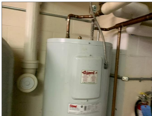
Non-asbestos fibreglass insulated hot water tank with metal jacketing.
