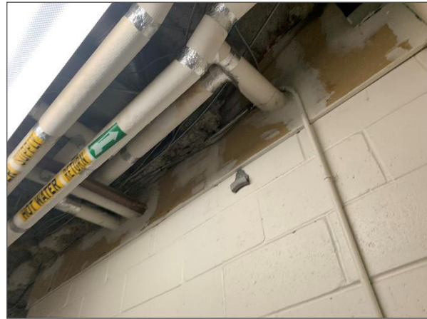
Non-asbestos fibreglass insulation.
