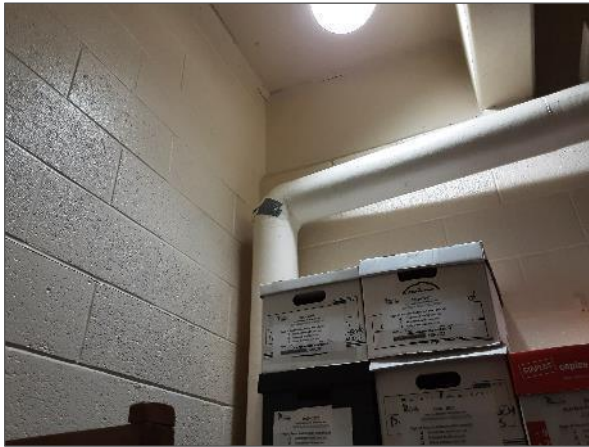
Asbestos-containing parging cement elbows and non-asbestos sweatwrap insulation.
