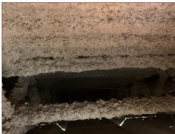
Non-asbestos spray-applied fireproofing.
