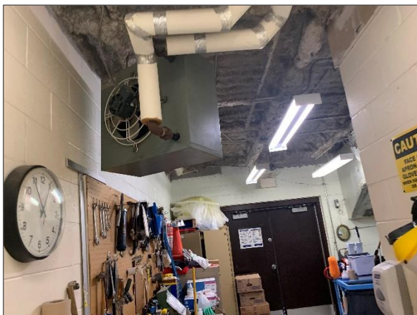
Uninsulated suspended unit heater.
